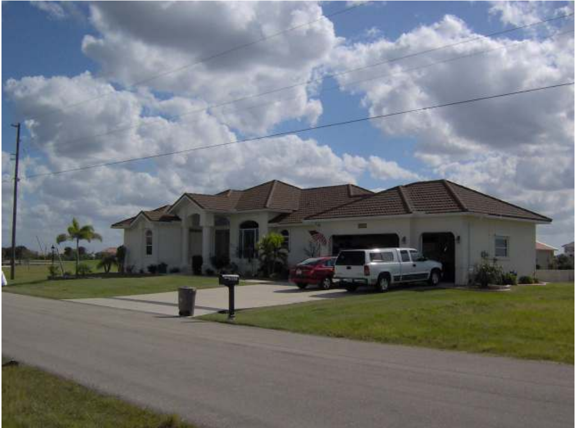
Figure B.3: Multiple Span Hipped Roof House
