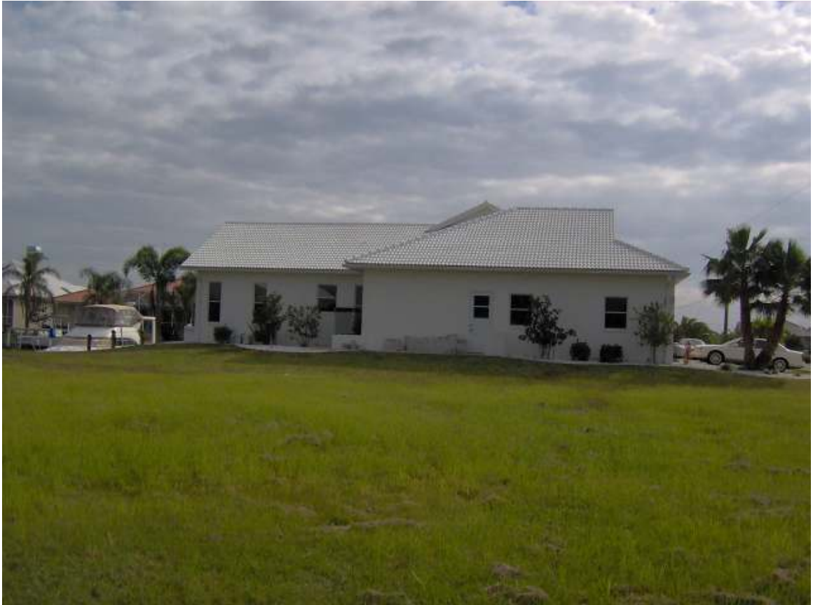
Figure B.5: Side View of a House that is Part-Gabled and Part-Hipped Roof
