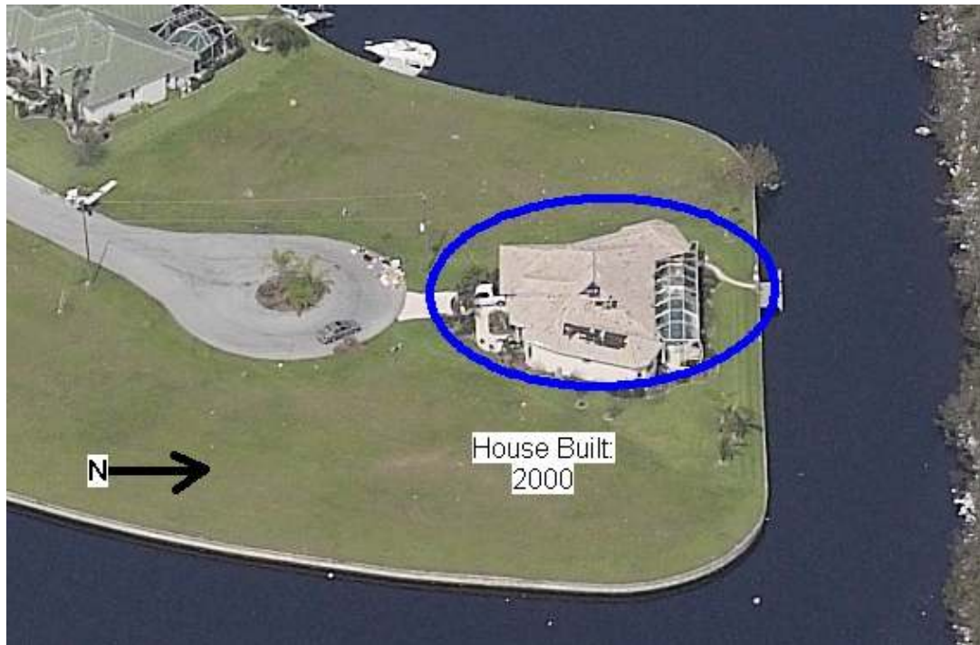
Figure A.8: Ridge and Corner Damage (Property #8)
