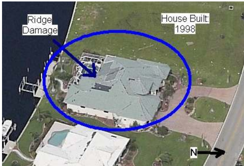
Figure A.20: Ridge Damage (Property #20)
