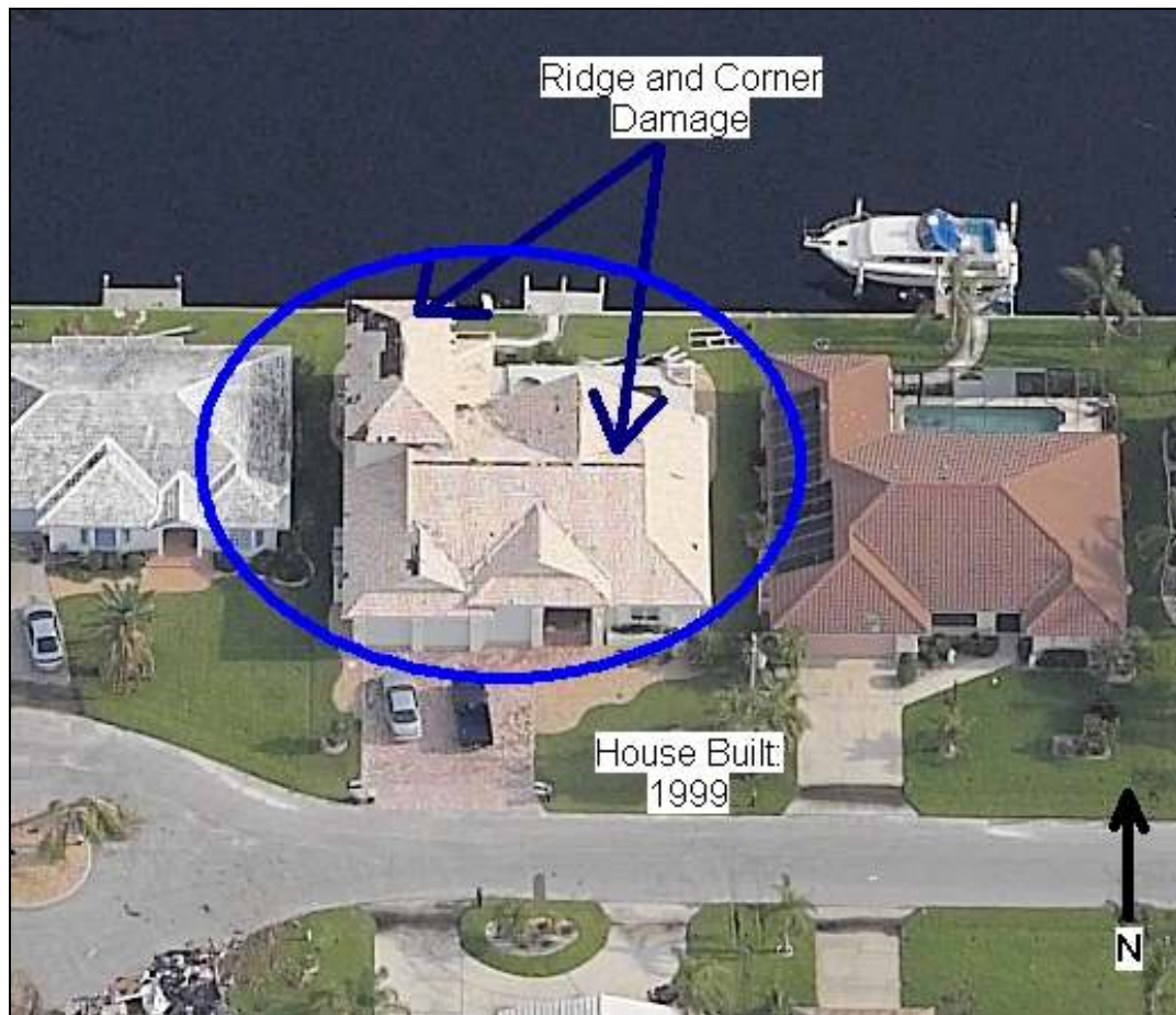
Figure A.3: Combination of Ridge and Corner Damage (Property #3)
