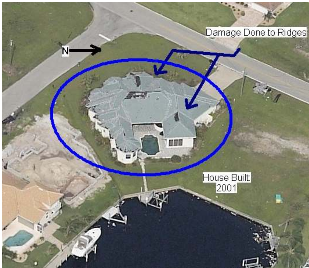
Figure A.13: Ridge Damage to a Large House (Property #13)
