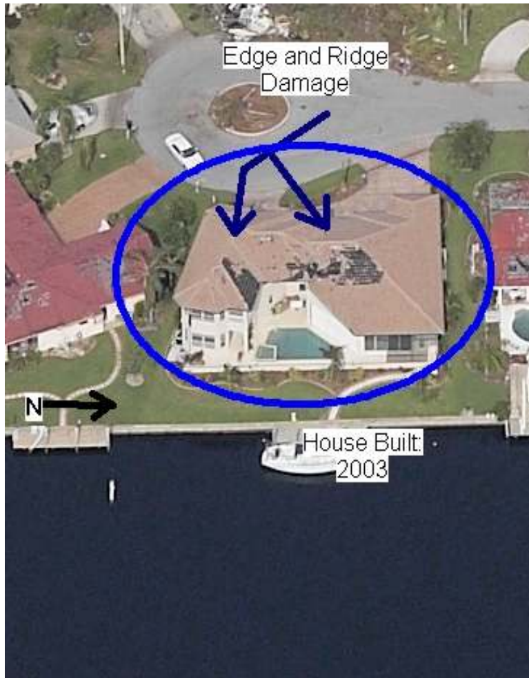
Figure A.22: Ridge and Edge Damage (Property #22)
