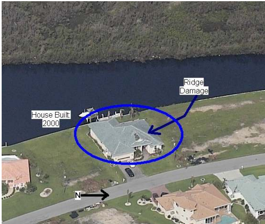
Figure A.15: Ridge Damage (Property #15)
