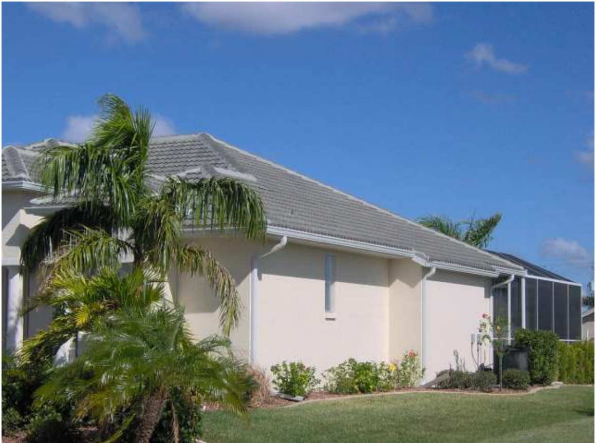
Figure B.2: View of the Wall of House #1
