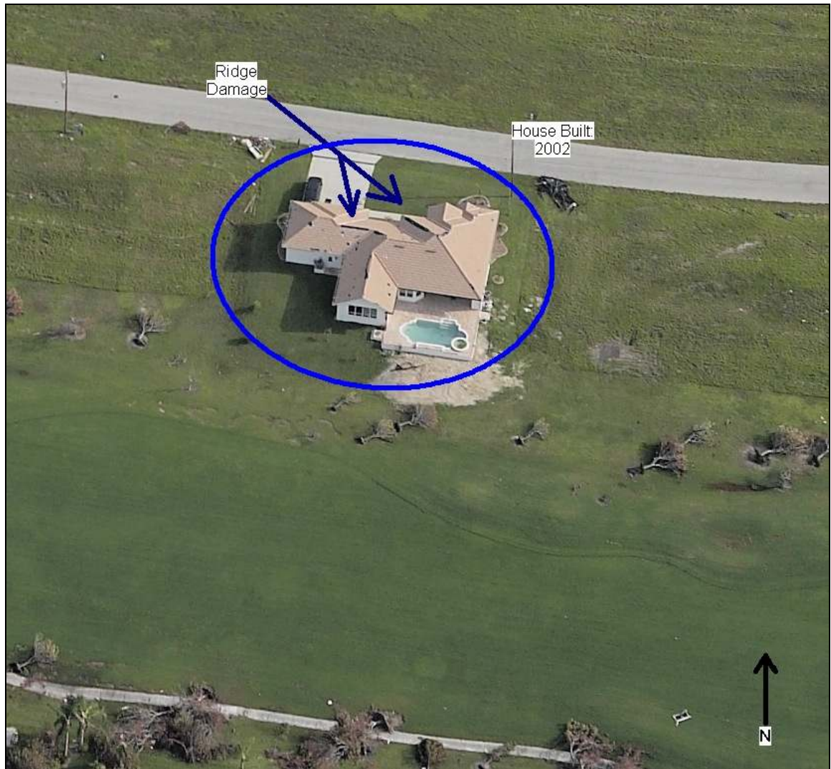
Figure A.1: Wind Damage Done to Ridges (Property #1)
