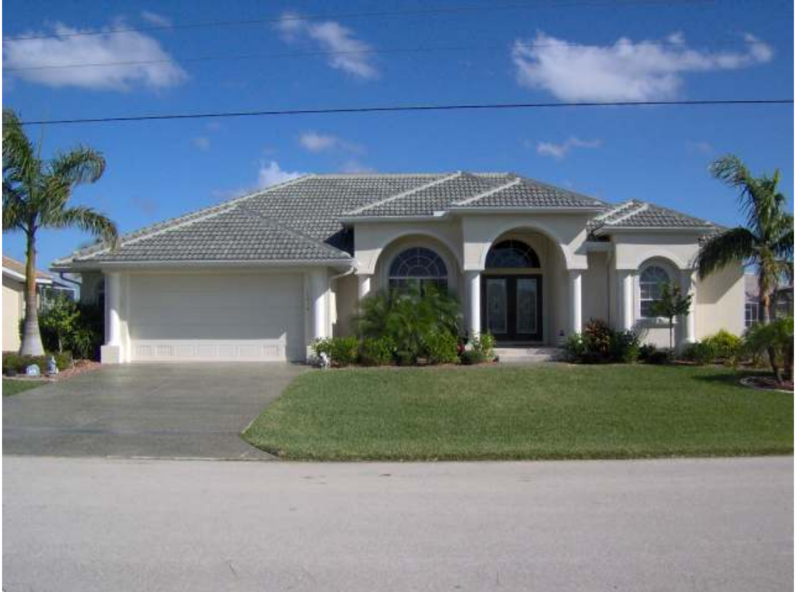
Figure B.1: Hipped Roof With Multiple Hips on One Span (Front View)
