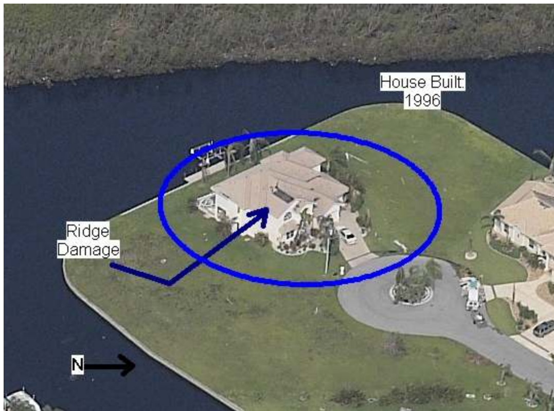
Figure A.16: Ridge Damage (Property #16)
