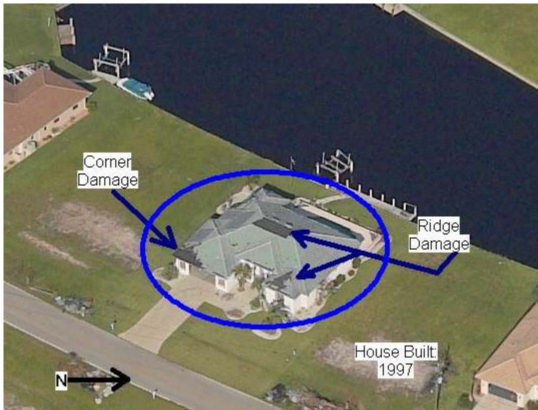
Figure A.14: Ridge and Corner Damage (Property #14)
