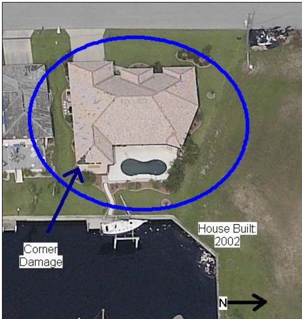
Figure A.6: Corner Damage (Property #6)
