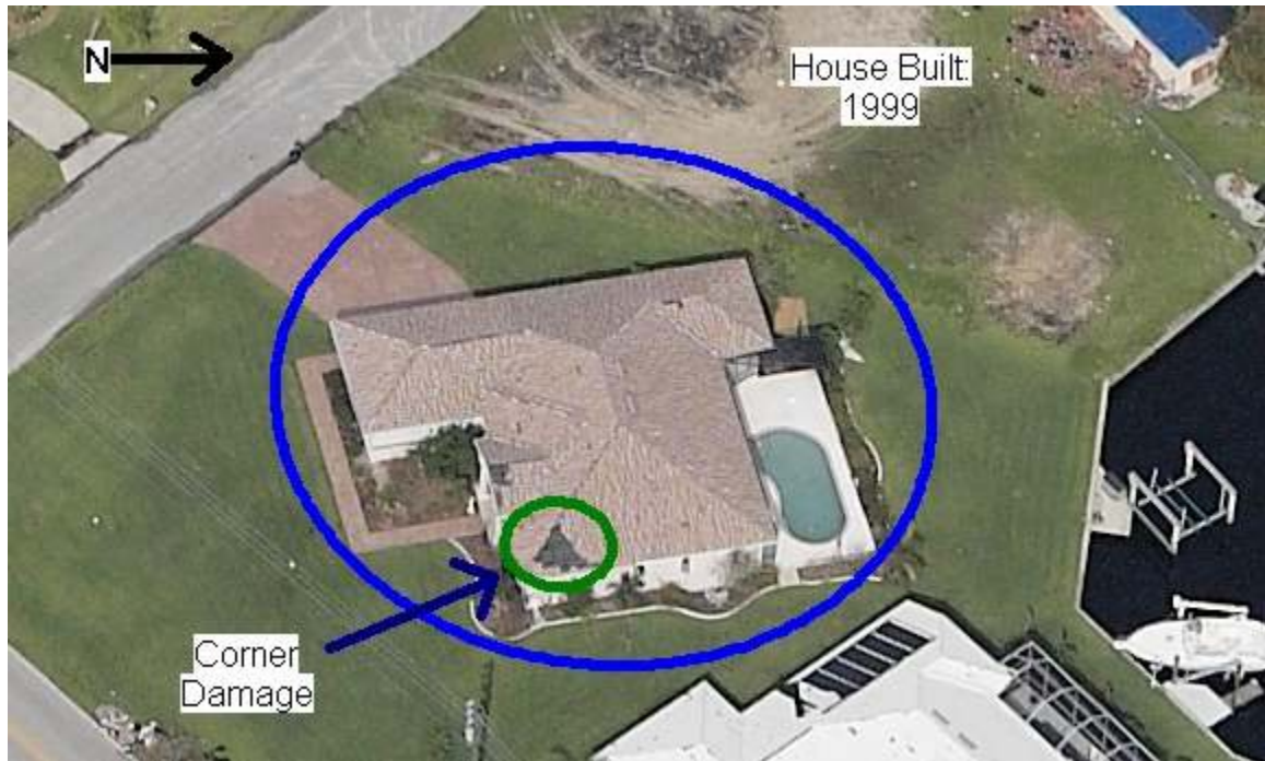
Figure A.12: Corner Damage (Property #12)
